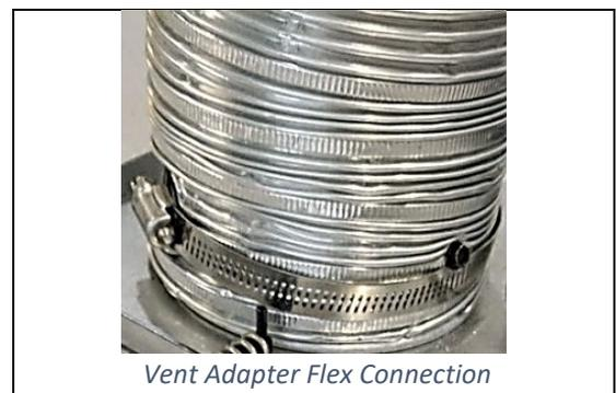
Once the two flex liners are dropped to the fireplace insert cavity, attach the 4" exhaust flex and the 4" air intake flex to the unit top vent adapter using hose clamps and sheet metal screws
